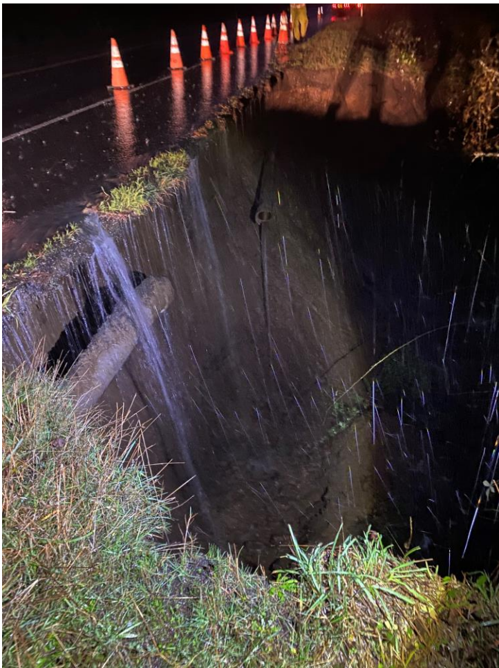
US HWY 101 – MP 145: December 20, 2021, looking South.
