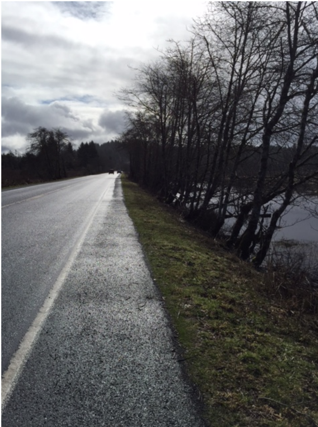
Photo 6. View of lane and shoulder width of west lane of N. Beaver Creek Road where the raw water pipeline would be located.
