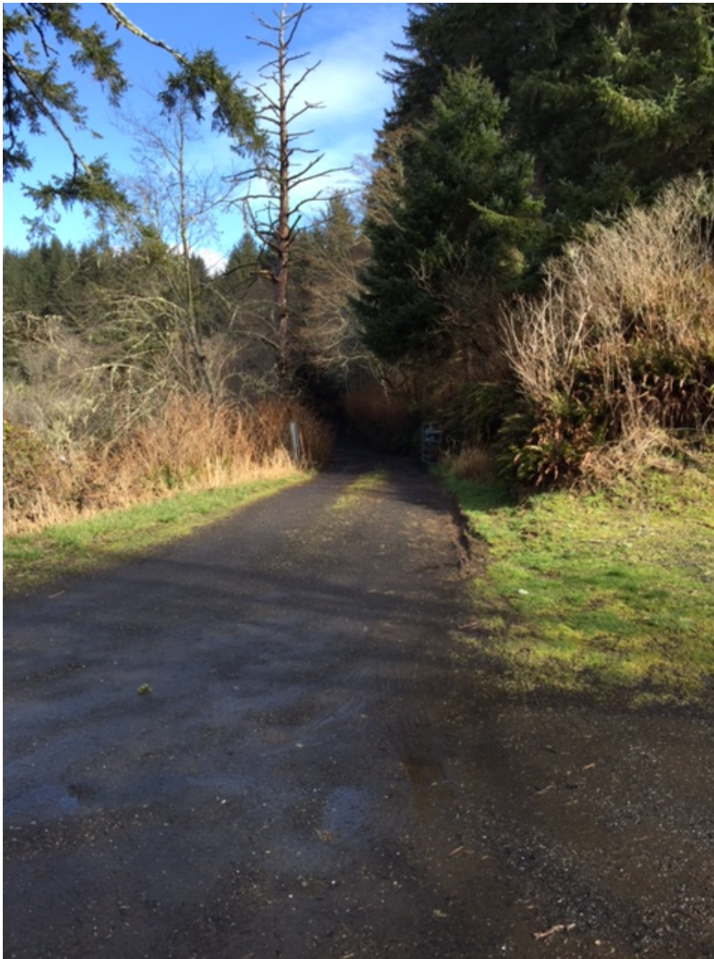
Photo 4. View of private road in which the raw water pipeline and backwash line would be run via trench uphill to the water treatment plant site.
