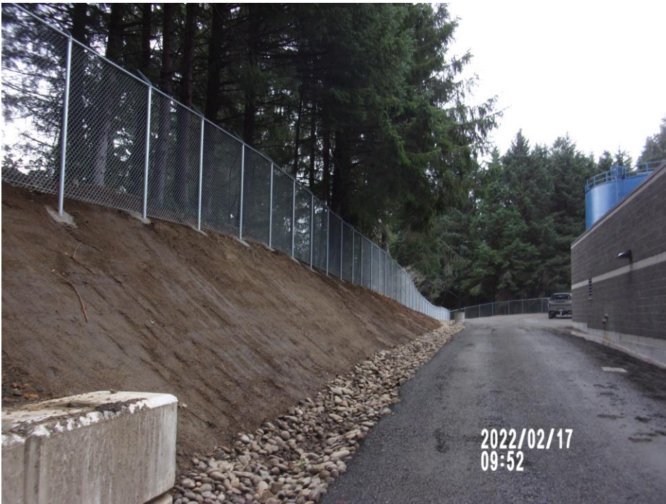
Onsite grading and fencing:
