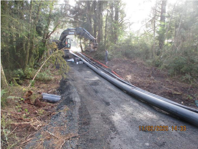
Pipeline placement towards Kona Place
