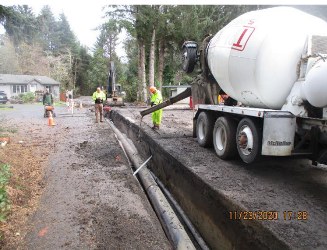
CLSM placement in pipeline trench at Kona Place
