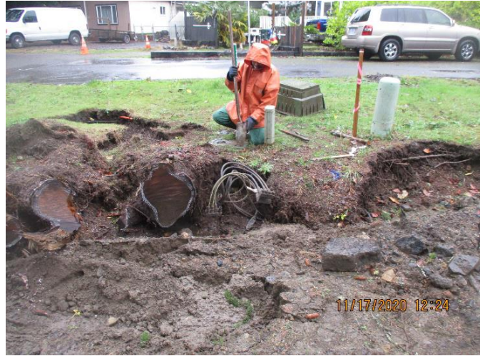
Existing utilities exposed on tax lot adjacent to Kona Place
