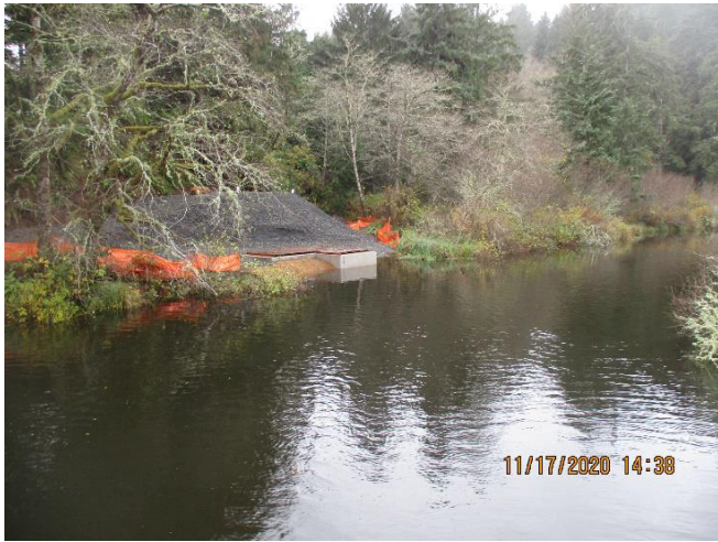
RW intake structure and surcharge loading – no activity in the month of November other than reestablishing BMPs
