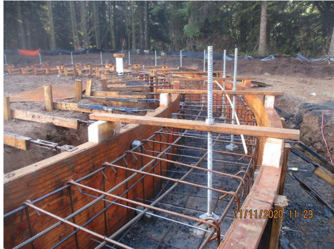
Anchor bolt and rebar placement for ringwall footing of Clearwell Tank
