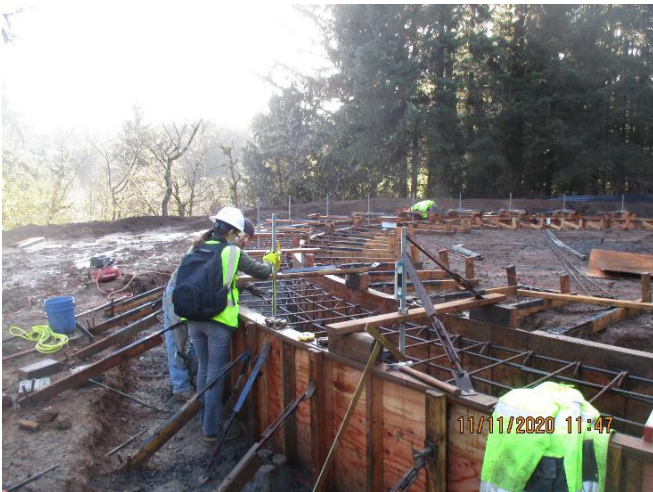
Structural observation of rebar and anchor bolt placement for Clearwell Tank
