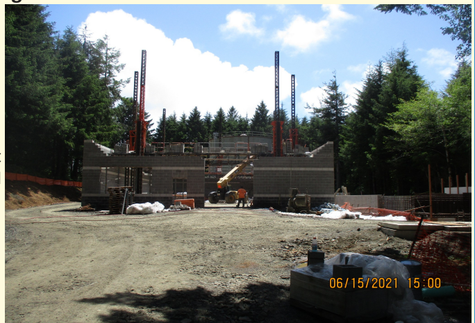
SRWD Membrane Treatment Building Under Construction
