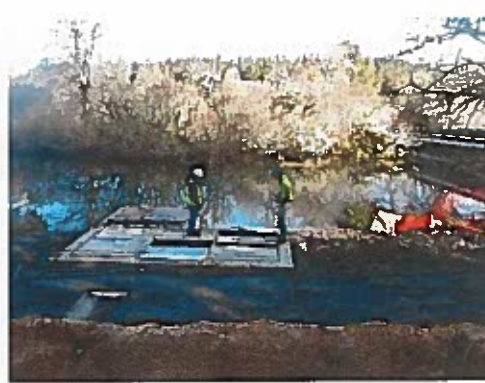
Intake with hatch covers:
