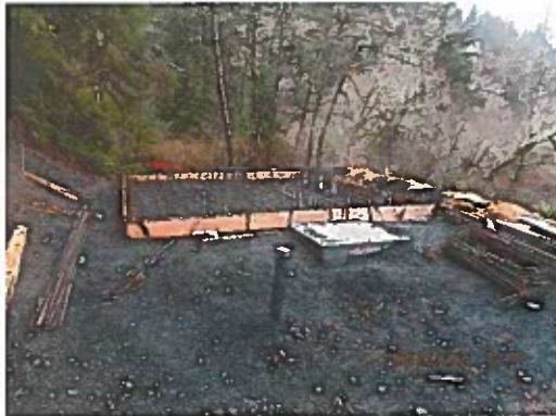
Intake Electrical Building pad:
