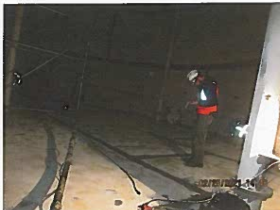
Interior of clearwell:
