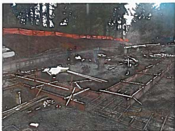
Membrane Building Footings:
