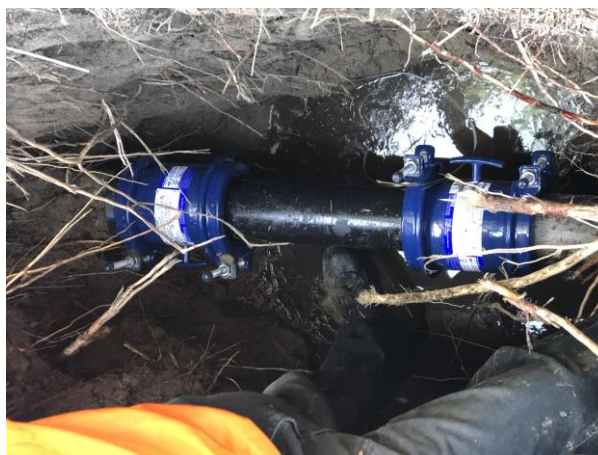
Temporary Repair June 26, 2019:
