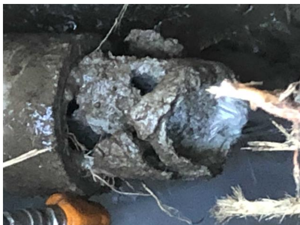
Canoe Street Waterline June 26, 2019:
