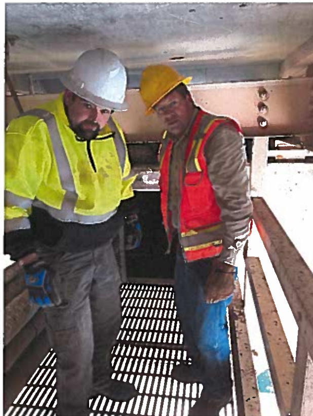
Exposed Access beneath the Alsea River Bridge:
