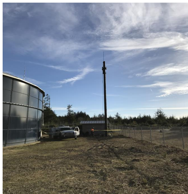
LOST CREEK AMI COMMUNICATION TOWER:
