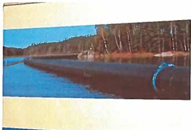
Olalla Reservoir Pipeline Crossing completed in 2016:
