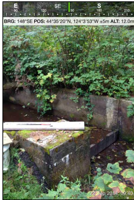
Weir and Overflow (Upstream View)
