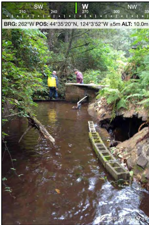
Existing Infrastructure Bank (Downstream View)
