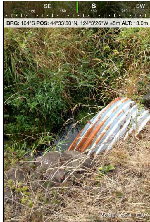
Culvert (Downstream View)
