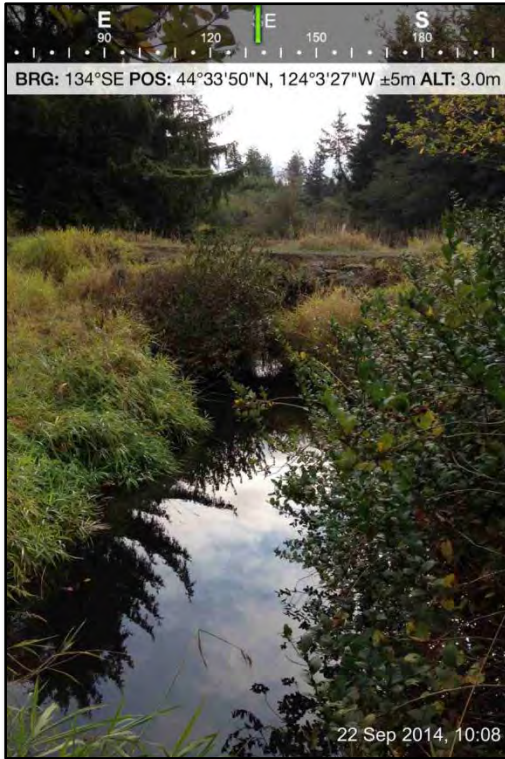
Culvert and Access Road
