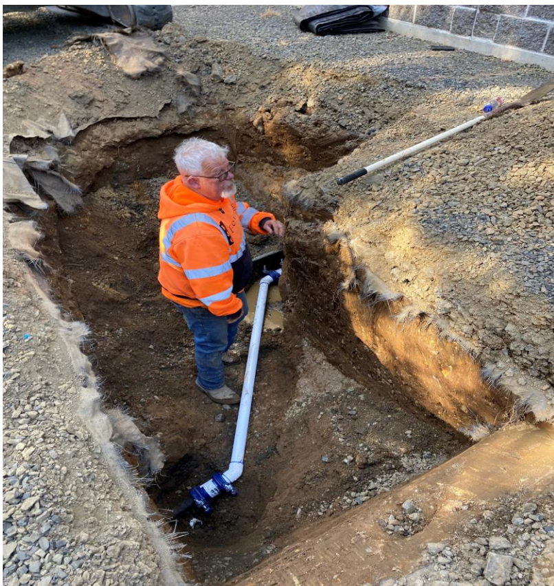
2-inch Drain Line Repair:
