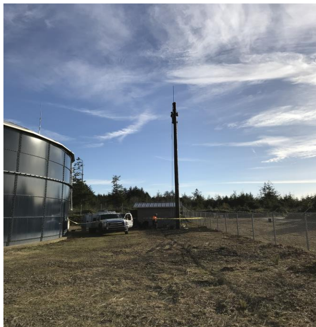
LOST CREEK AMI COMMUNICATION TOWER:
