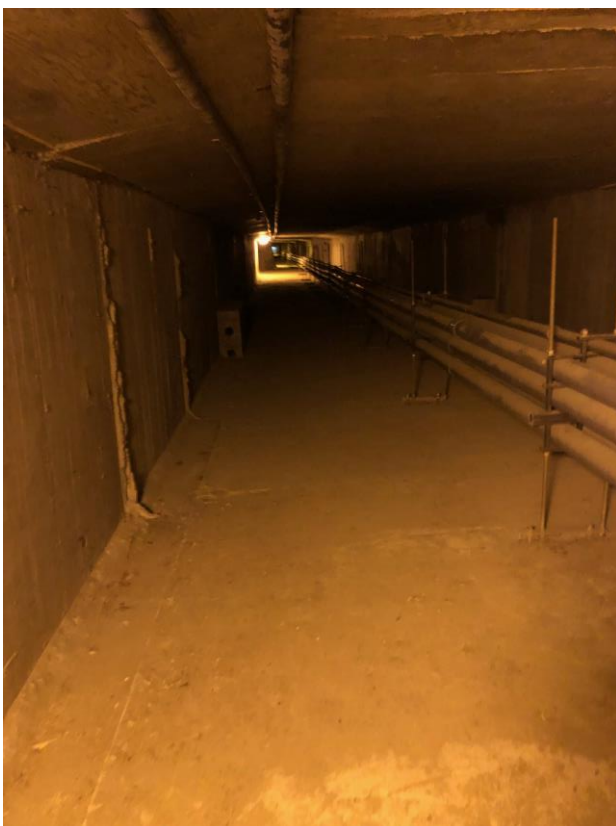
Enclosed Access beneath the Alsea River Bridge:
