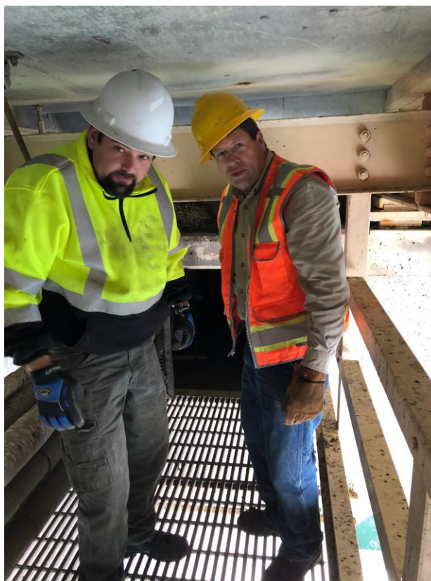
Exposed Access beneath the Alsea River Bridge:
