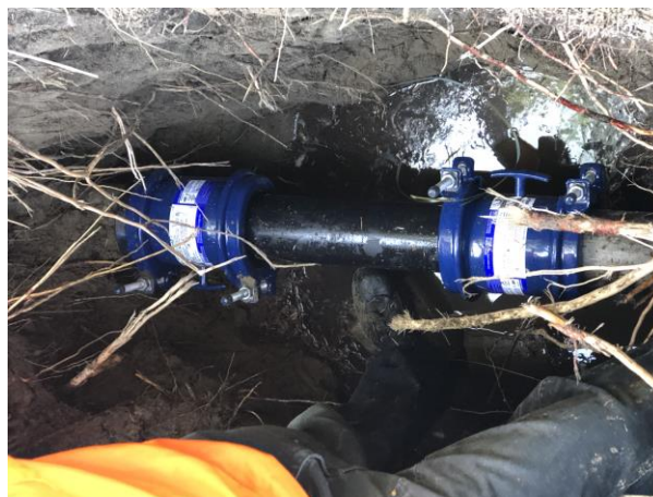
Temporary Repair June 26, 2019:
