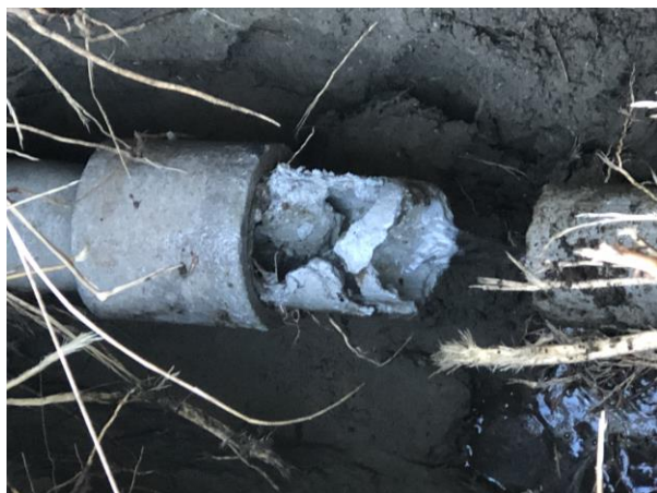
Cano Street Waterline June 26, 2019:
