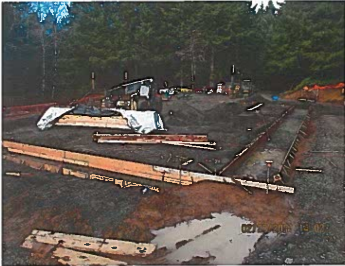
Membrane Building footings:
