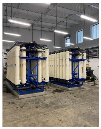
Water Treatment Plant (WTP) Operators continue working with Jacobs Engineers and the membrane filter skid provider, WesTech to improve operational performance at the water treatment plant. Filter skids are using much less power and chemicals during the clean in place (CIP) process and operators are recognizing much longer run times between CIP's.
