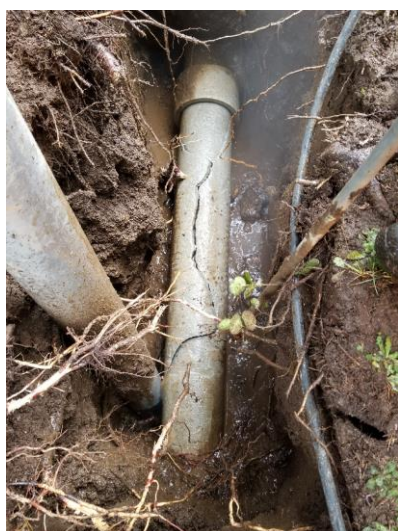
Ruptured pipe 01/16/2019:
