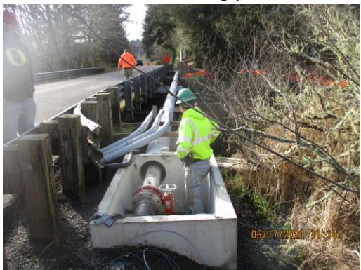
Bridge piping north vault:
