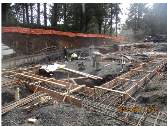
Membrane Building Footings:
