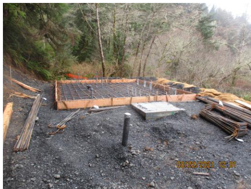
Intake Electrical Building pad:
