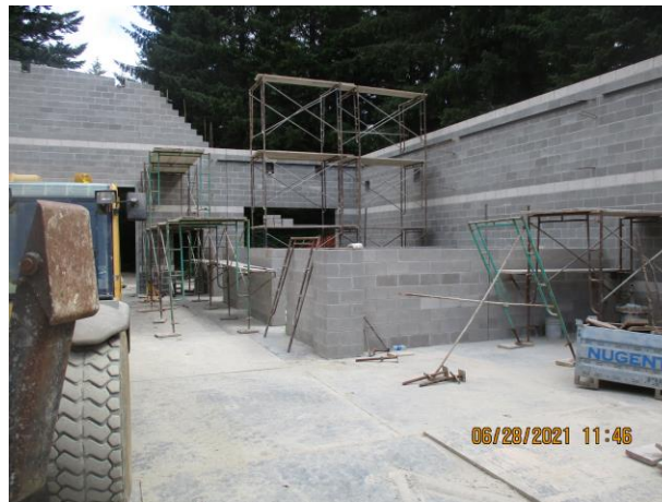
Membrane Building Block Wall Construction:
