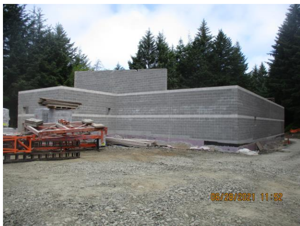
Membrane Building Block Wall Construction:
