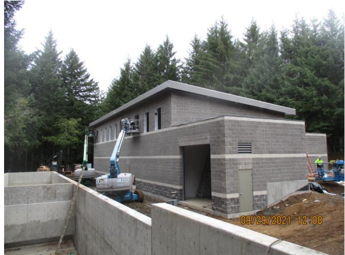
WTP window installation:
