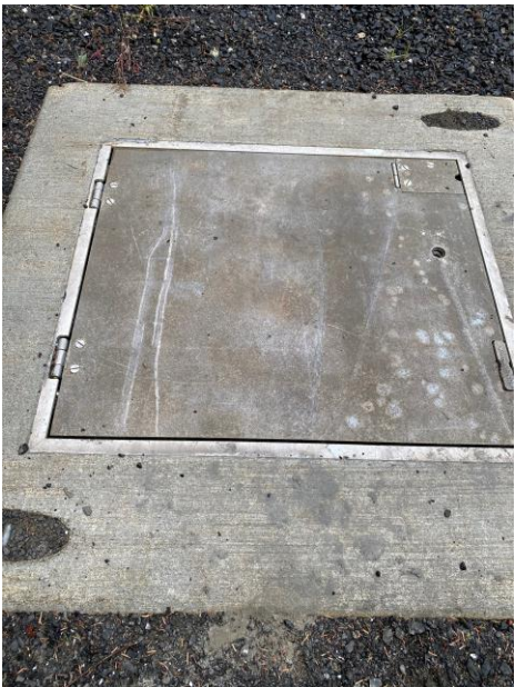
Damage to Intake Hatch Doors:
