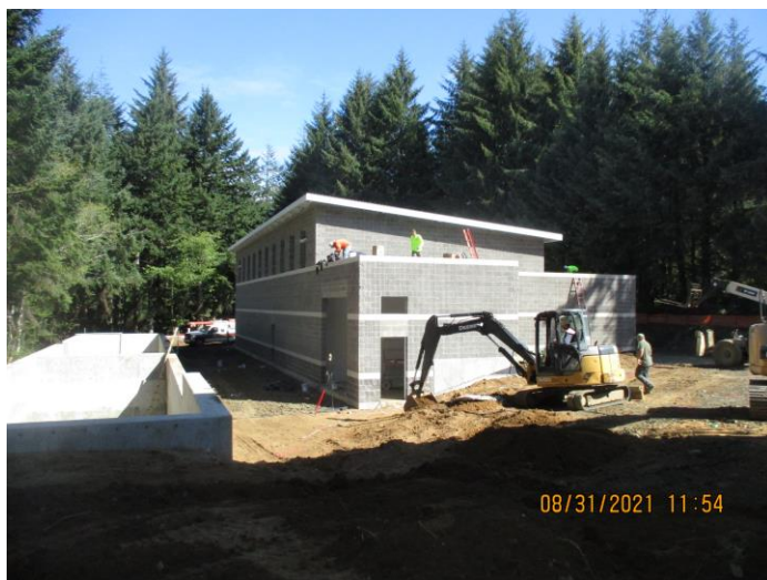
Completed Backwash Basin:
