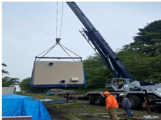
123 rd Street Pump Station:
