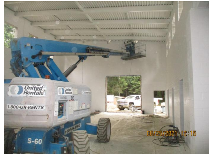
Interior painting Membrane Building:
